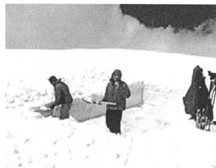
Clearing the site for work
